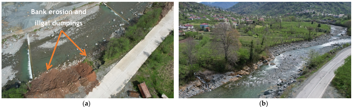
Figure 11. Illegal dumping of (a) dirt and rubble into Sidere Creek next to the roads and (b) a perspective view of a lower part of the study area. The images were captured by the DJI Air 2S drone.
