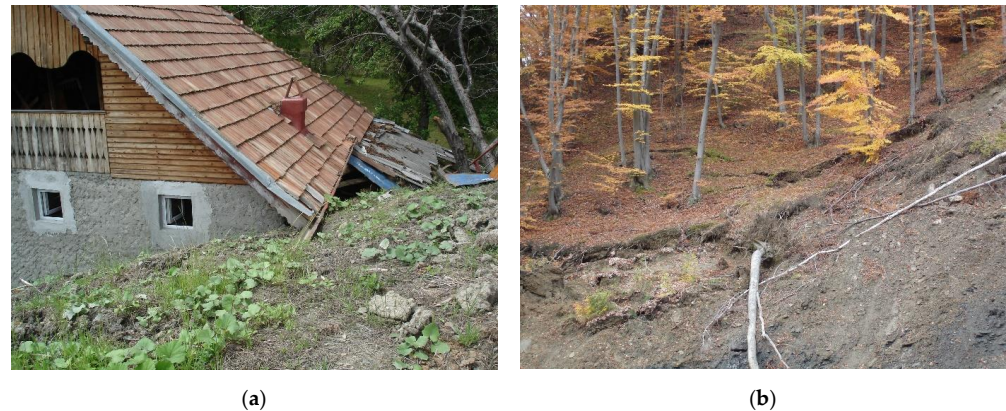
Figure 16. The impacts of the Chirlesti mudflow (a) in an urban area where soil covered the building up to the roof; (b) forested area along the streambank that collapsed.
