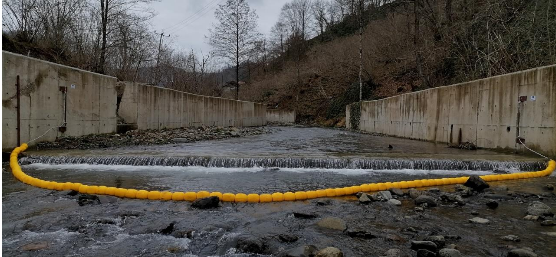
Figure 1. Litter Trap in Stream; design to capture floating litter in stream flow.
