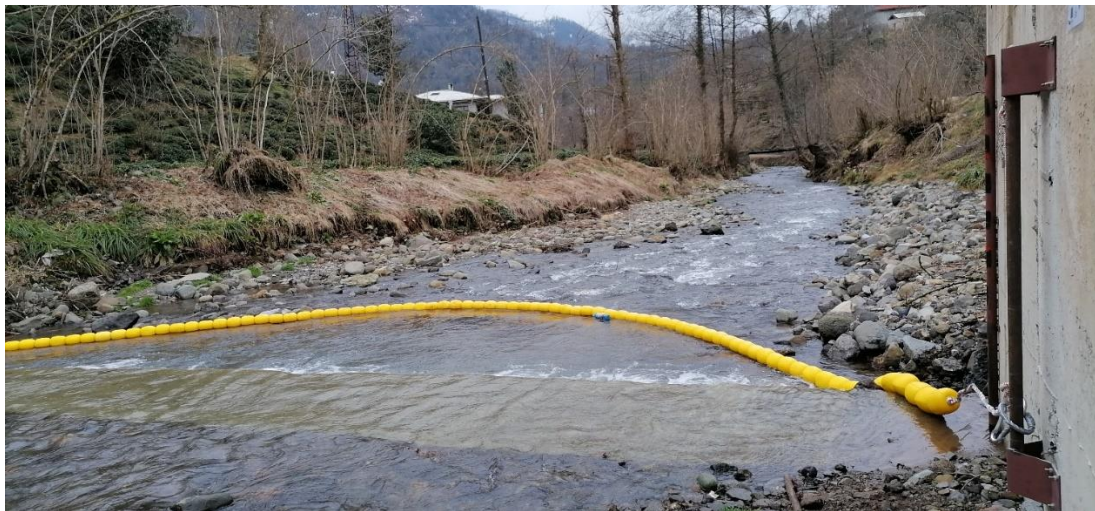
Figure 2. Litter Trap and It's Mechanism that allow it raise during high flow
