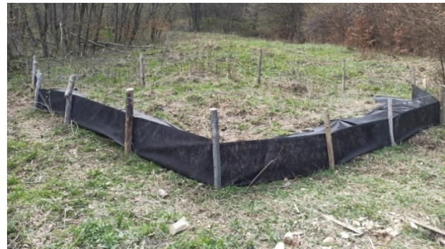
Fig.2. Alluvial trap installed
